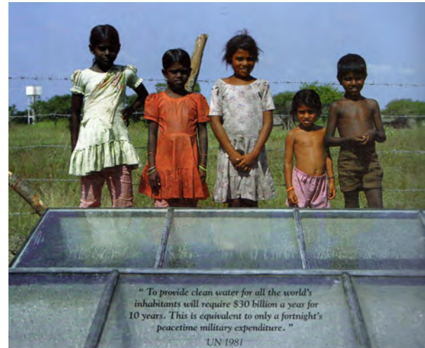
Solar desalination plant. Sri Lanka. A Suntec Foundation project.
