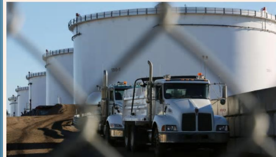
Kinder Morgan's North 40 terminal expansion construction project near Edmonton, Alberta, 2016. © Reuters
